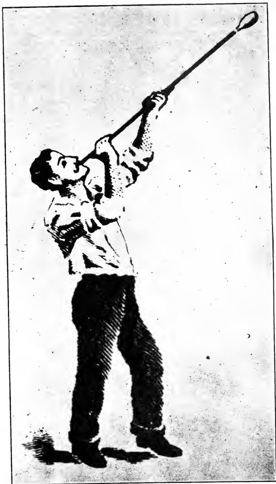
FIGURE 1.—Glass blower at work. Illustrates bottle-making methods prior to 1905.
